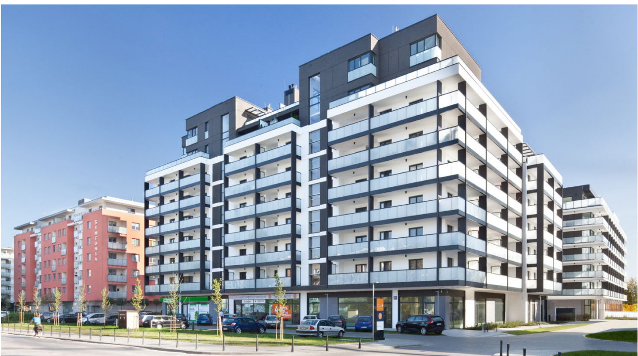
„Miesto Wola” Residential Estate in Warsaw
